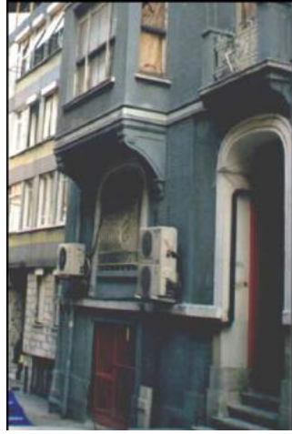
Figure 13. Ground floor use of Bilsak Building, Soğancı Street, 2001.
