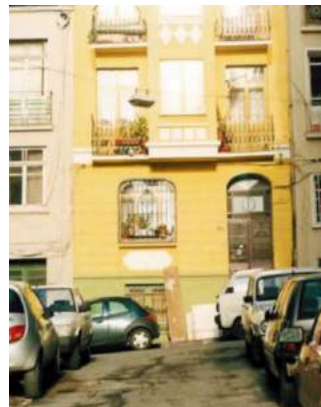
Figure 17. Matara Rise, asphalt surfacing, 2001.
