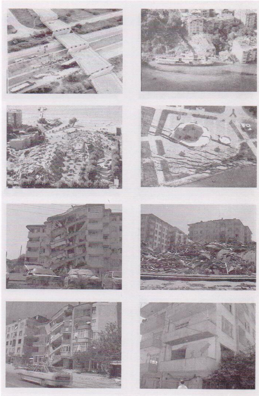
Figure 2. Views after the Kocaeli earthquake
