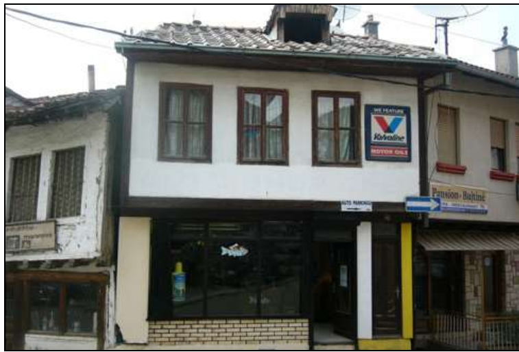
Figure 48: Traditional buildings in two-story heights
