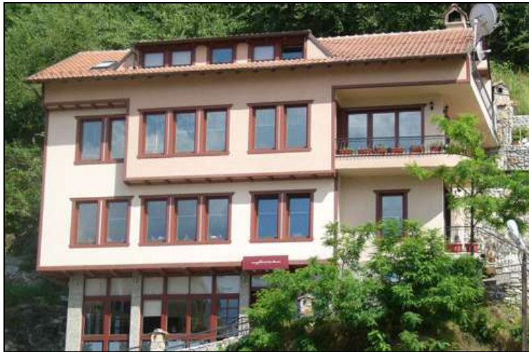
Figure 45: Building in good condition
