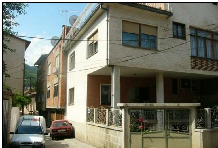
Figure 58: Building in disharmony
