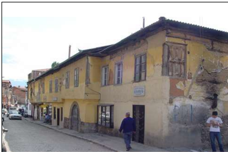
Figure 46: Building in bad condition
