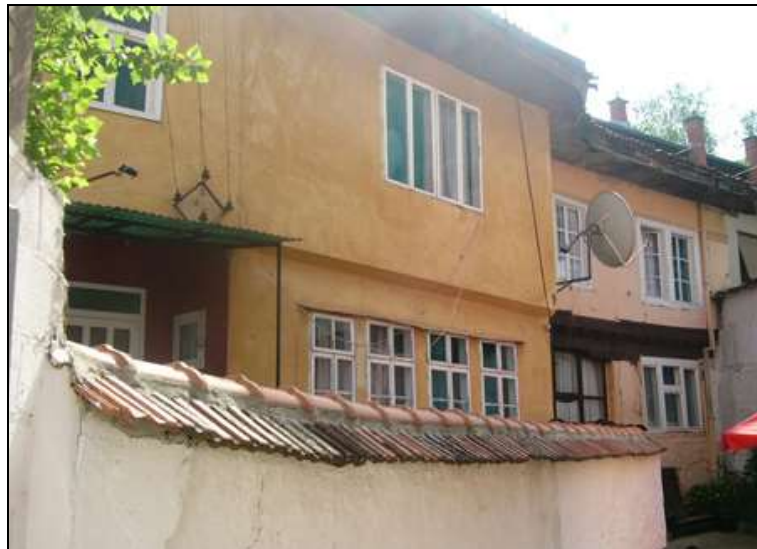
Figure 52: Building in masonry
