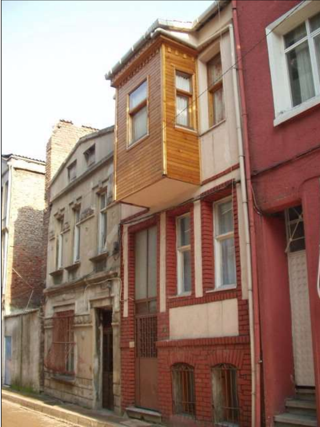
Figure 26. Building in Good Condition
