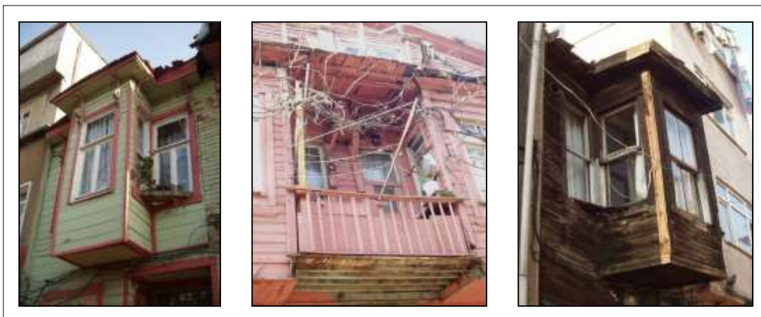
Figure 33. Bay Windows of Listed Buildings
