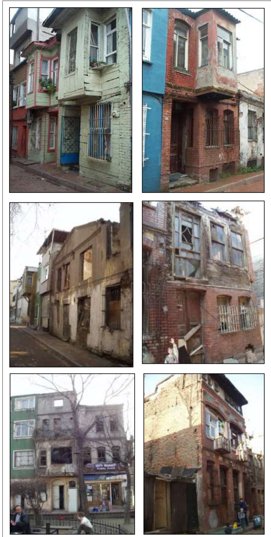
Figure 23. Buildings in Bad Condition
