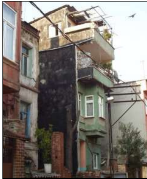
Figure 39. Building in Disharmony
