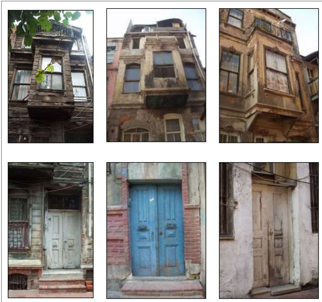
Figure 32. Doors of Listed Buildings
