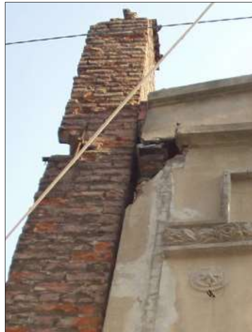
Figure 52. A Listed Masonry Structure in Yenikapı
