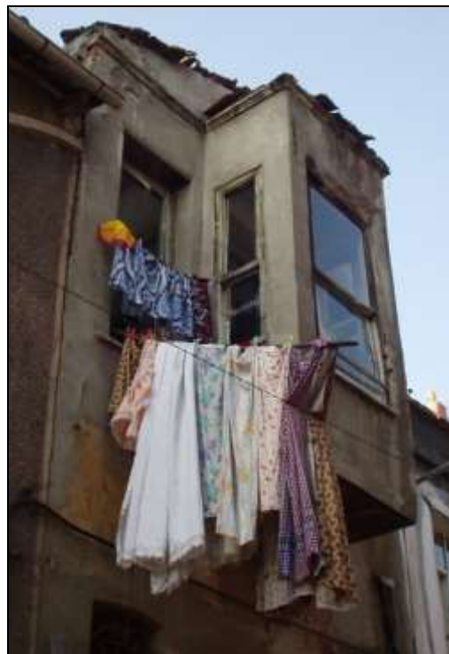
Figure 51. A Listed Masonry Building
