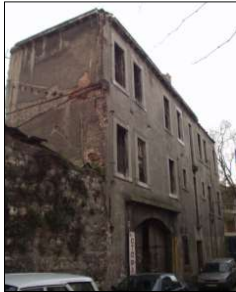
Figure 32. An Unoccupied Listed Building
