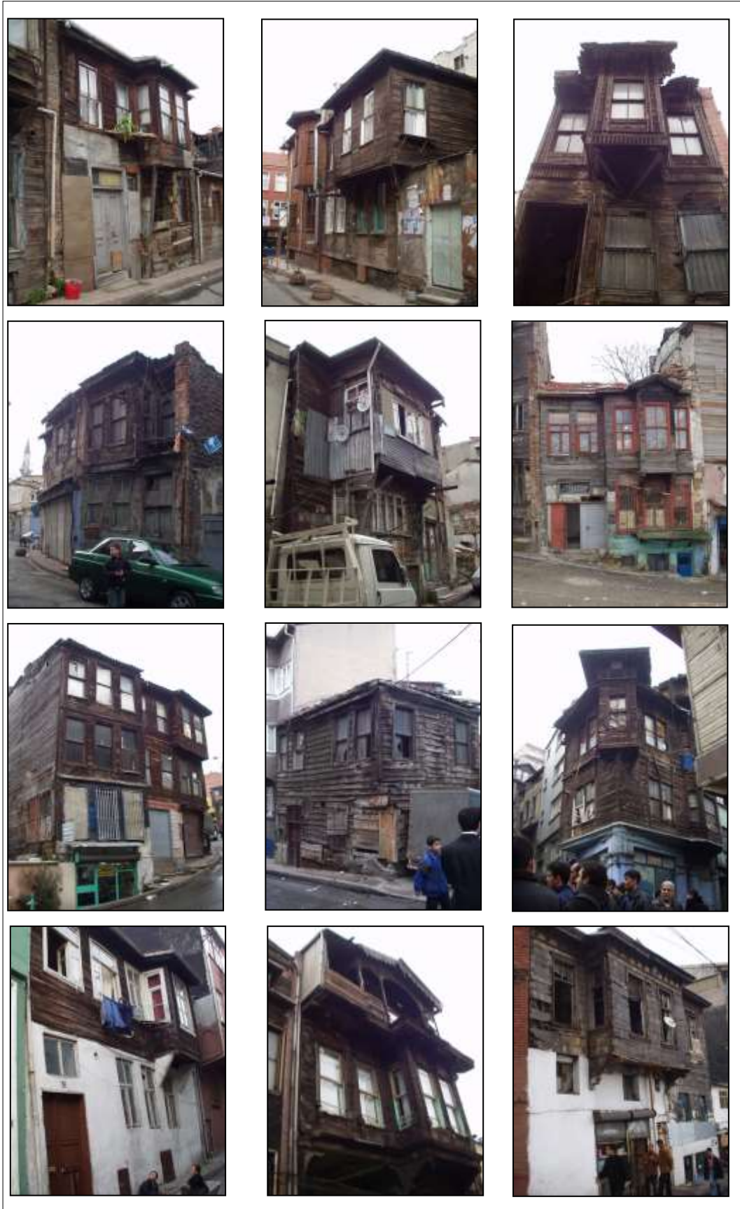
Figure 26. Listed Timber Buildings
