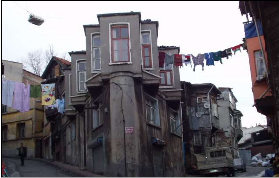
Figure 28. A Listed Masonry Building
