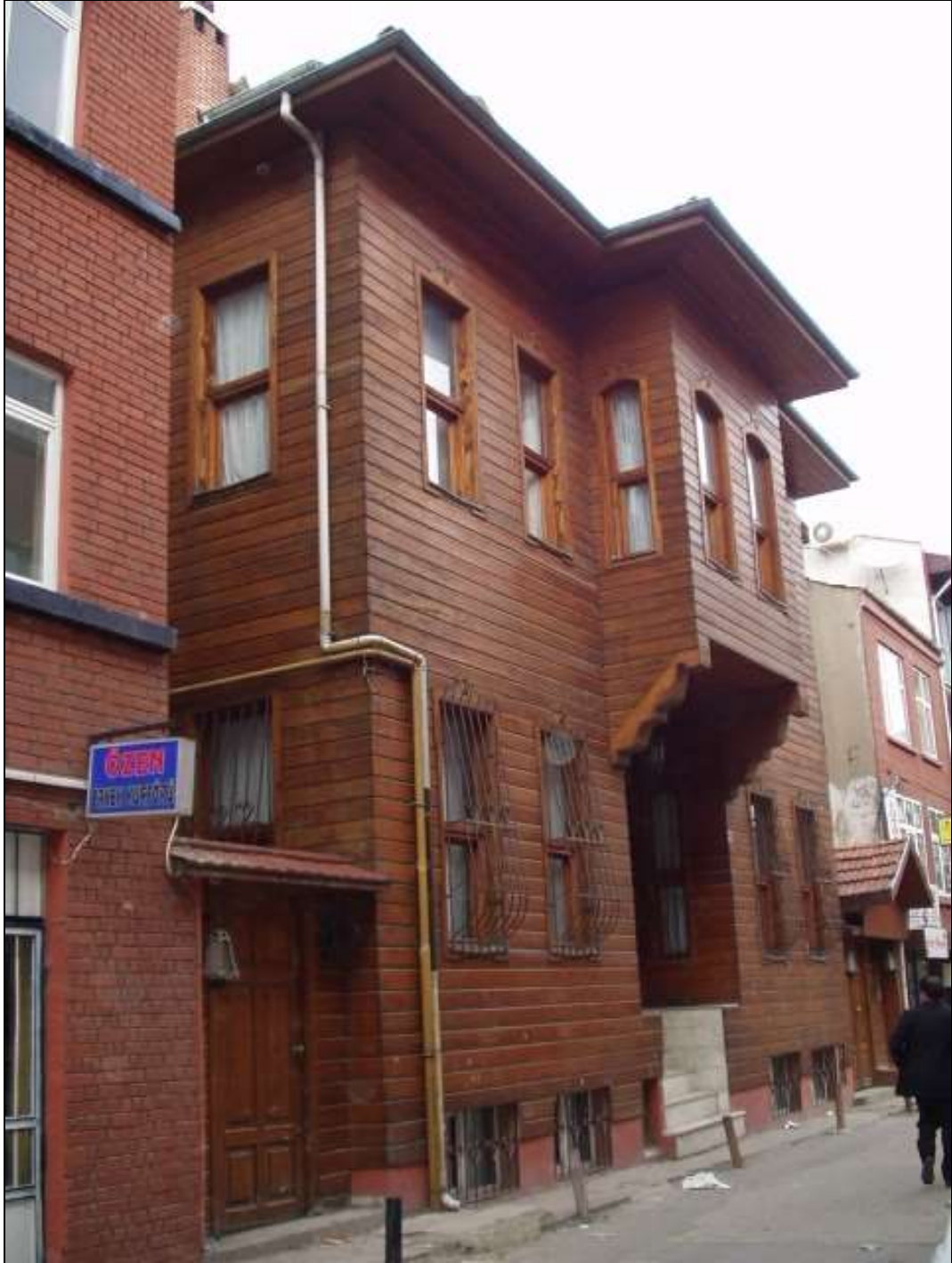
Figure 47. A Timber Building in Good Condition
