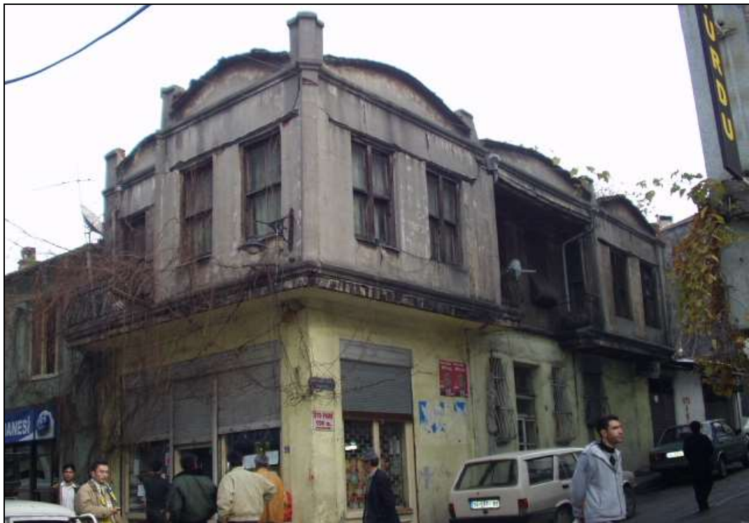
Figure 29. Listed Masonry Building
