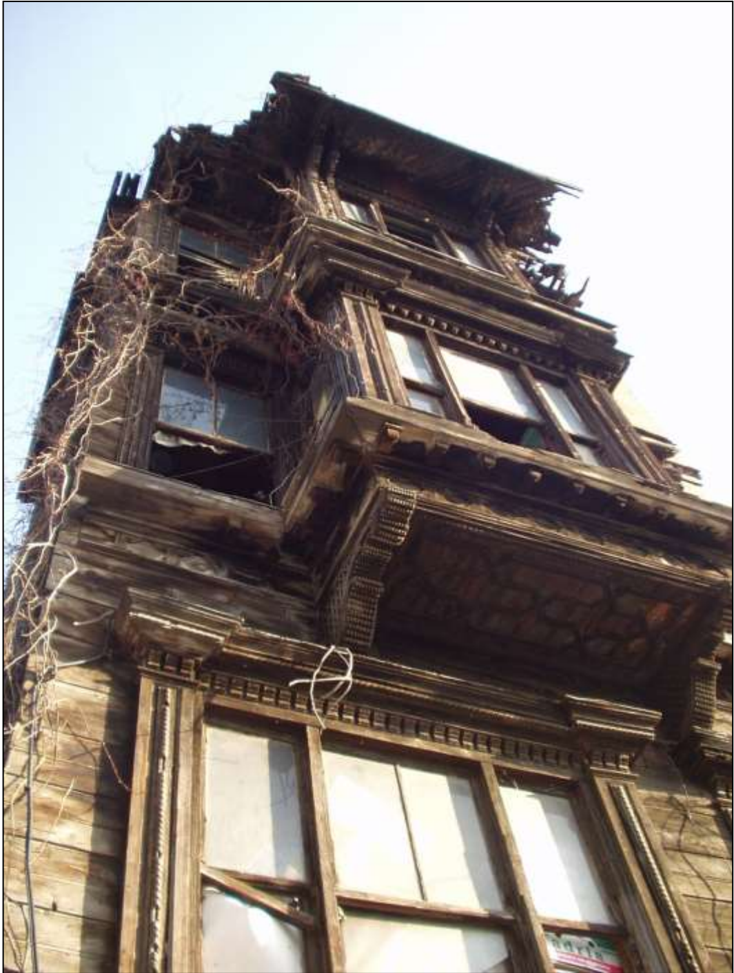
Figure 45. Timber Building in Detail
