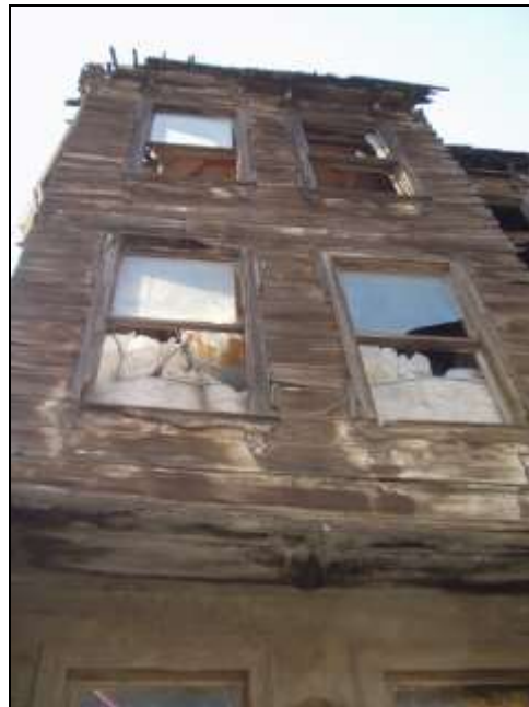
Figure 33. An Unoccupied Listed Building
