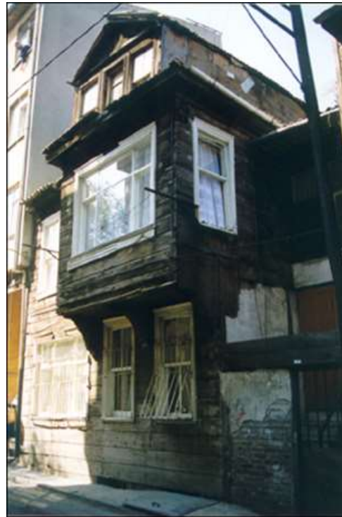
Figure 59. Timber Building Having Intervened Façade
