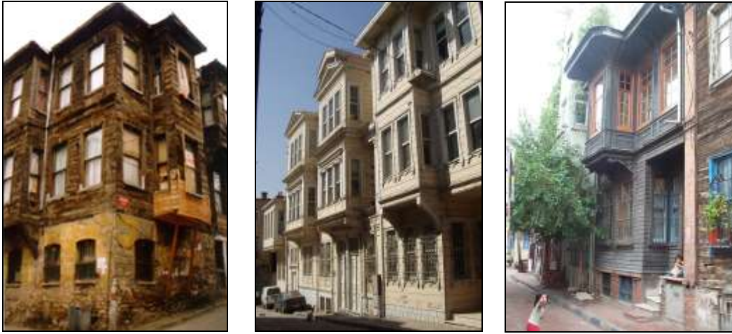
Figure 47. Listed Timber Structures in Zeyrek, Süleymaniye and Yenikapı
