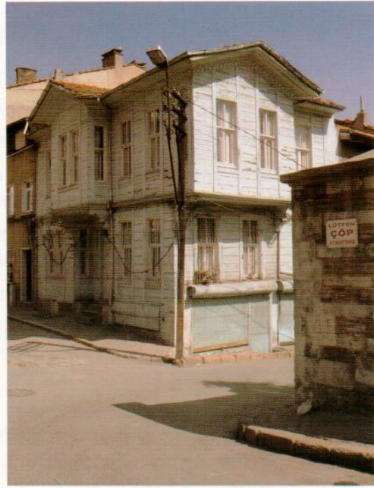
Figure 7. Civil Architecture in Zeyrek
