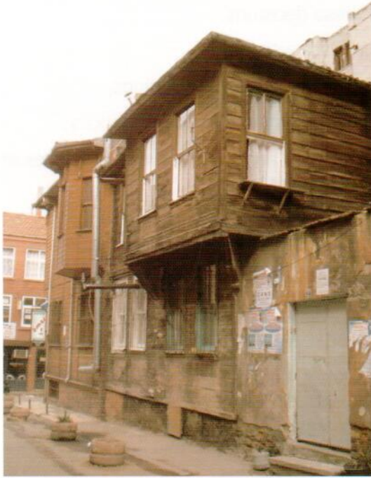
Figure 6. Civil Architecture in Zeyrek
